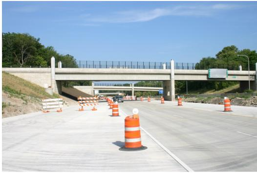
FAI Route 74 (WB) from Nebraska Avenue to Monroe Avenue, including 10.8 m and variable width continuously reinforced concrete pavement, two at 3.0 m width concrete shoulders, drainage work, retaining walls and bridge work.
